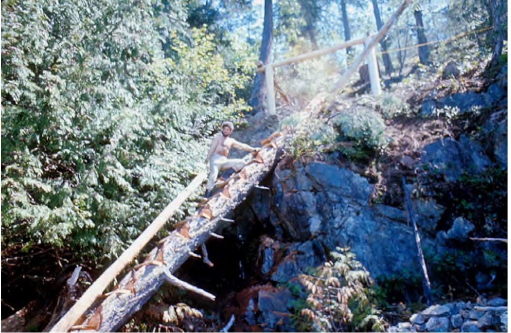
The twin log staircase made it easier to haul up building logs.
